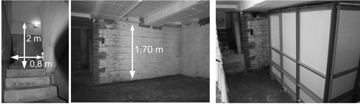
Fig. 4: Integration of a storage (4,2 m 3 ) in a residential building: Limited access (left), low room height (middle), installed storage with an optimal use of available room.
