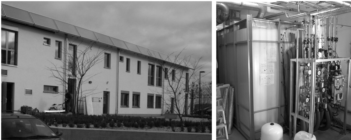
Fig. 5: Installed Modular buffer storage (Company Wagner & Co. Solartechnik, Kirchhain, Germany)
