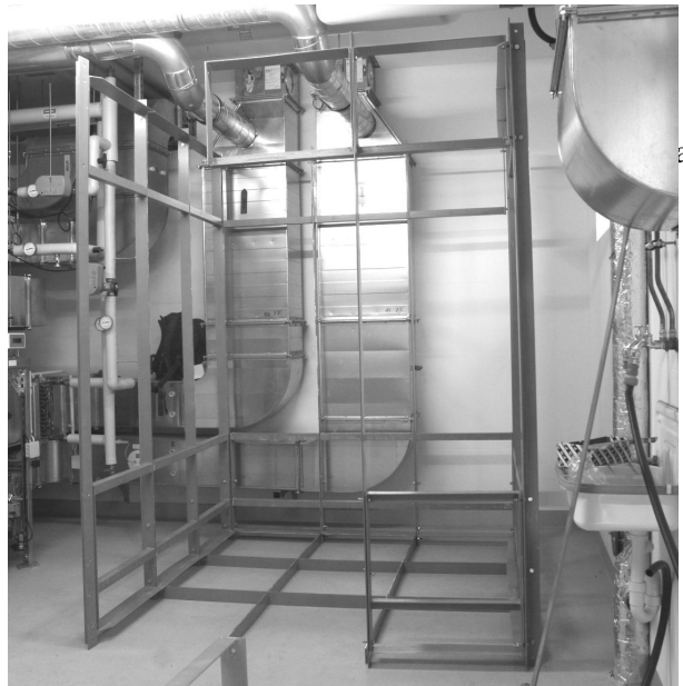
Fig. 3: Steel frame construction of the modular storage, partly assembled
